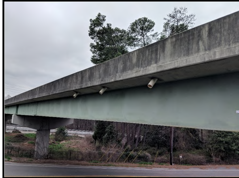
6 PVC scuppers were observed during the assessment of the bridge.
